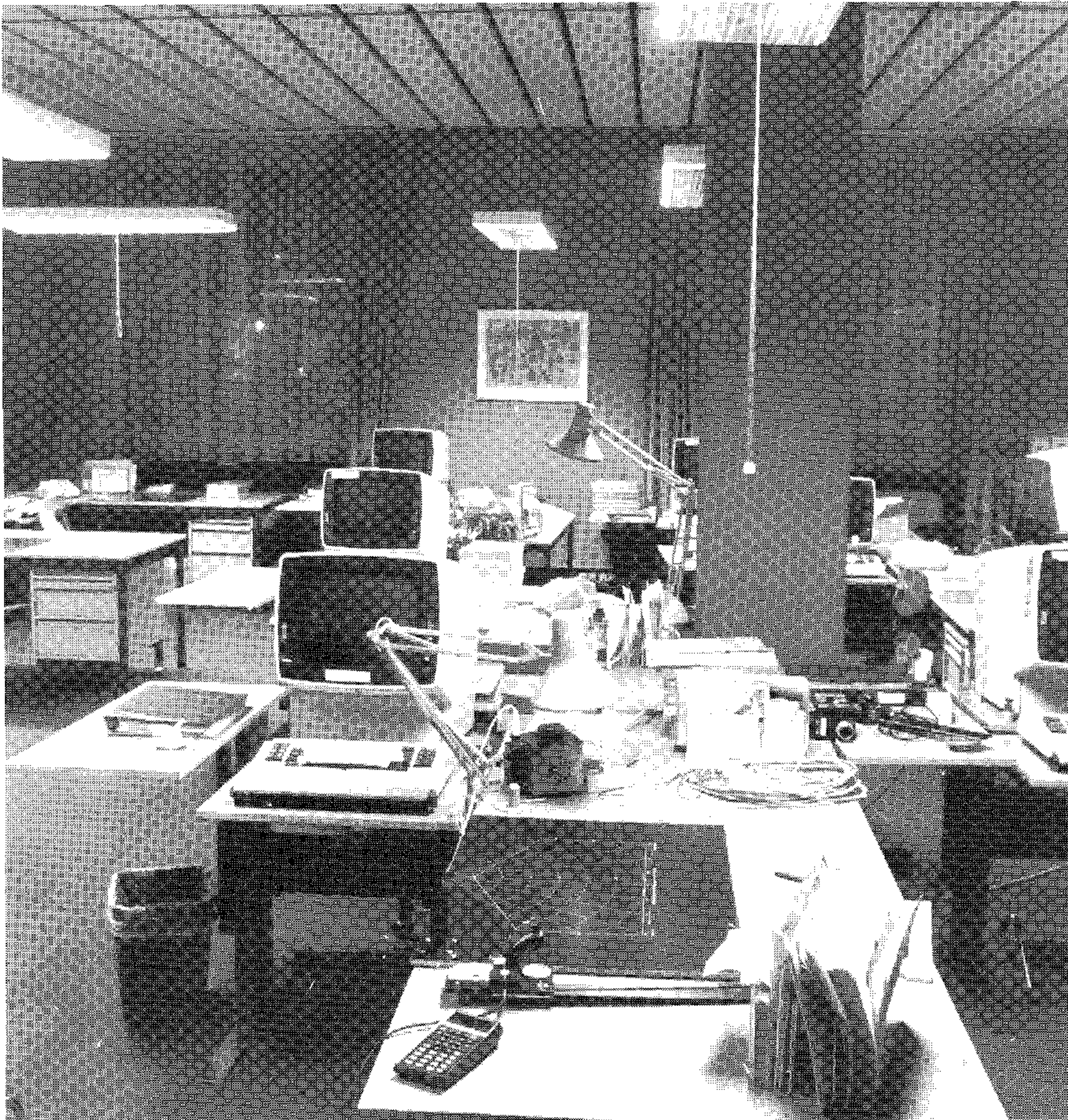
Fig. 23. An example of luminaires with low luminance louvres enabling the effects of reflections and glare on the screens to be avoided. On the other hand, the luminaires are too widely spaced to give a good contrast rendering on the desks: a localised lighting at each workplace is necessary.
