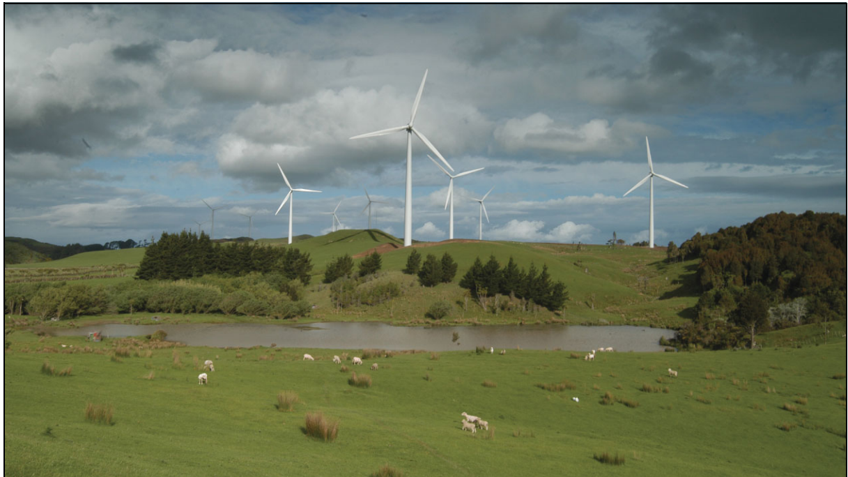
Fig. 1 The site as it will look after the commissioning of the wind farm
