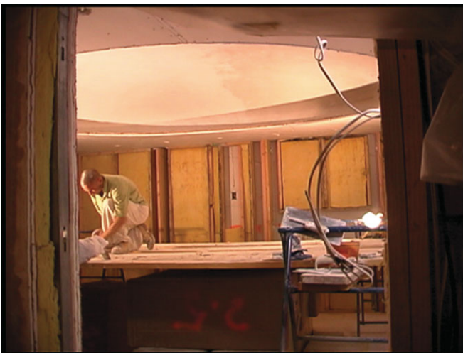
Fig. 4 Left: Elliptical lath and plaster dome, under construction. The combination of the specialized (porous) acoustical plaster material, support structure and damped air cavity above makes for an effective, broadband absorber. The interior wall cavities (stud bays) are being fitted with varying densities of fibreglass absorbents to attenuate transverse waves Right: Side wall as acoustically transparent fabric is stretched into place. Yates employs a Brüel & Kjær Falcon™ Range 1/2-inch Microphone Type 4189 in a custom-built chamber to test the acoustic transparency of wall and ceiling fabrics under consideration
