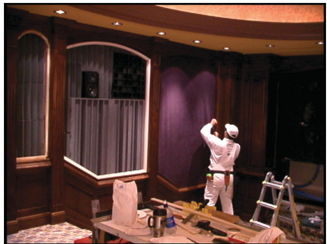
Fig. 4 Left: Elliptical lath and plaster dome, under construction. The combination of the specialized (porous) acoustical plaster material, support structure and damped air cavity above makes for an effective, broadband absorber. The interior wall cavities (stud bays) are being fitted with varying densities of fibreglass absorbents to attenuate transverse waves Right: Side wall as acoustically transparent fabric is stretched into place. Yates employs a Brüel & Kjær Falcon™ Range 1/2-inch Microphone Type 4189 in a custom-built chamber to test the acoustic transparency of wall and ceiling fabrics under consideration
