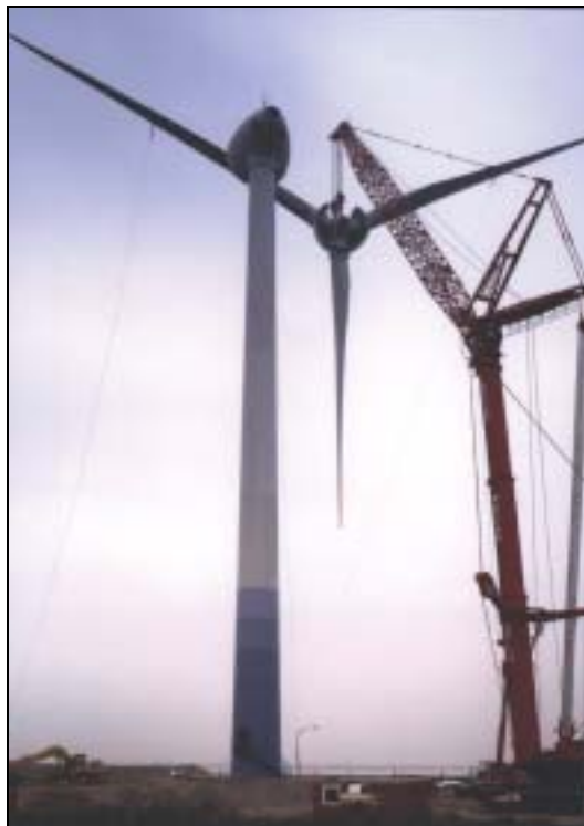
Fig. 6 A Liebherr crane hard at work
